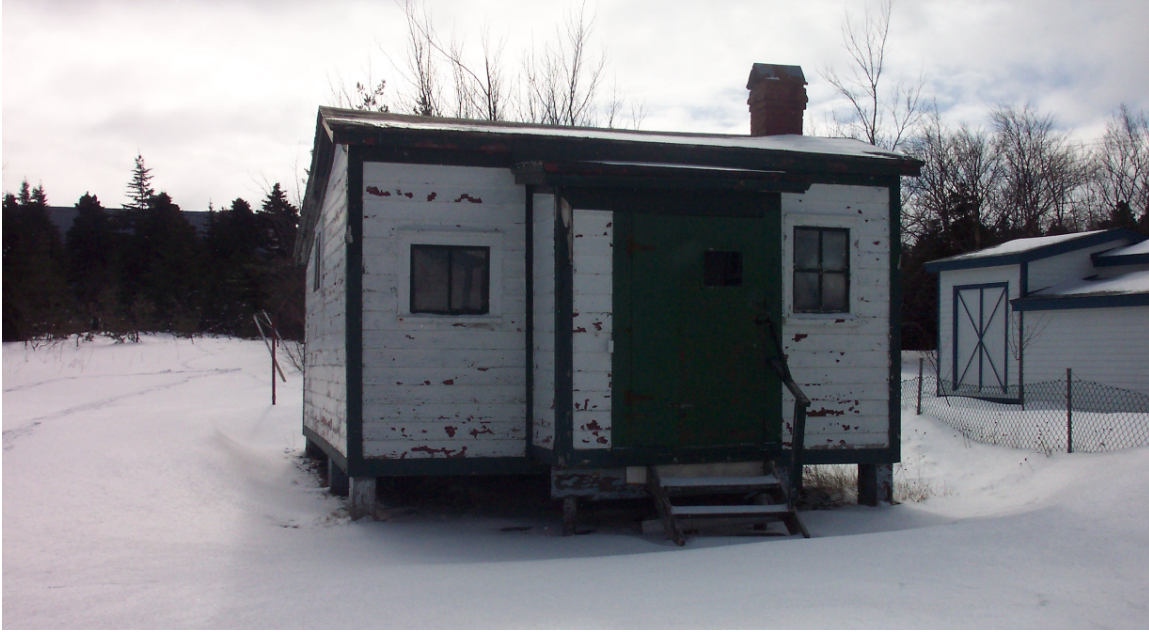
Stan Percy's Cottage, 167 Park Avenue, First Phase of Construction, 1937.
