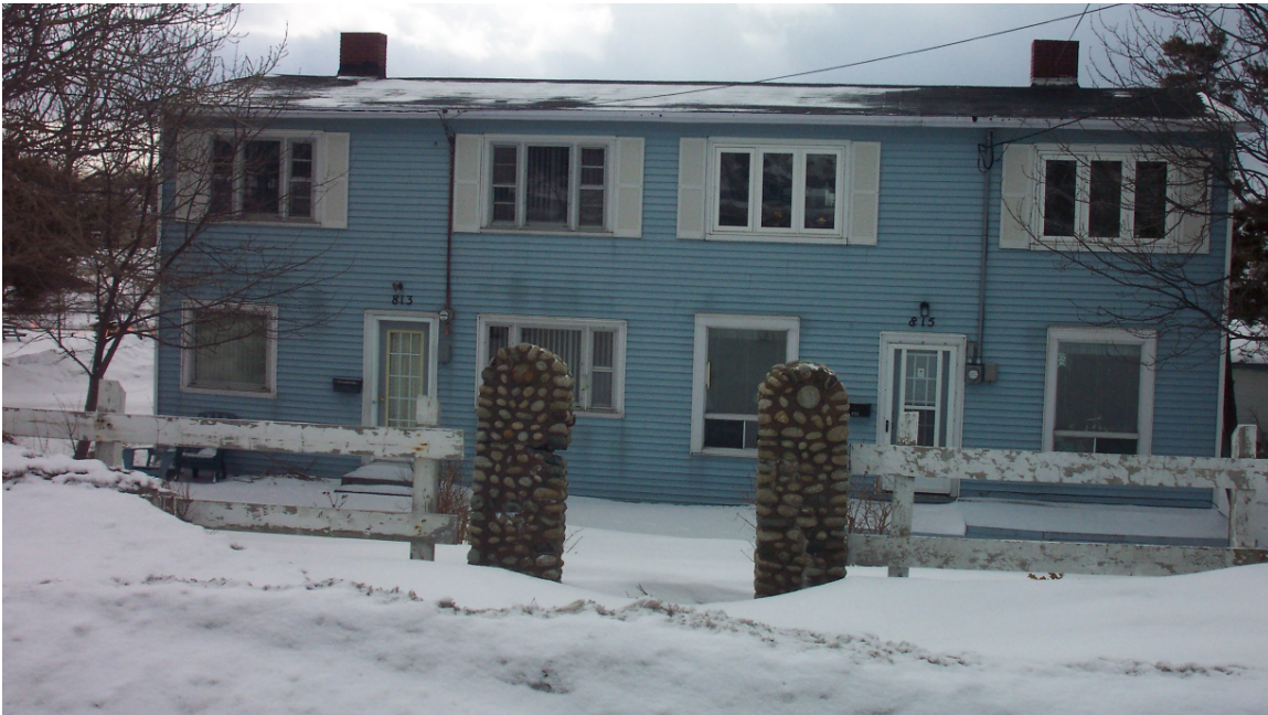
813-185 Topsail Road, front view, February, 2005.
