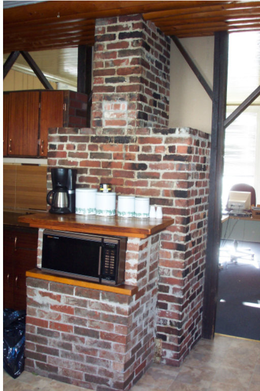
Kitchen hearth, 906 Topsail Road. Front brick section may have been added.
