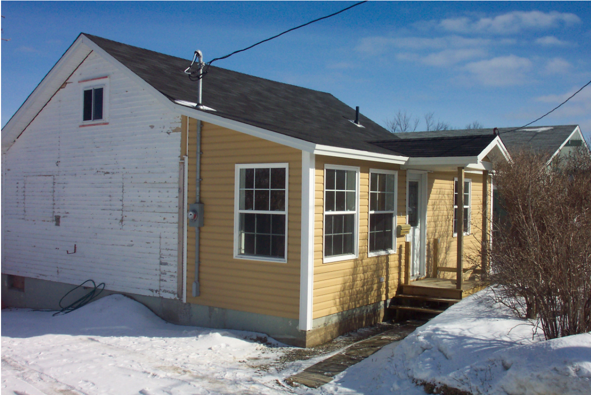
204 Park Avenue, February, 2005. Note new windows and vinyl siding in front, compared to narrow clapboard in back.
