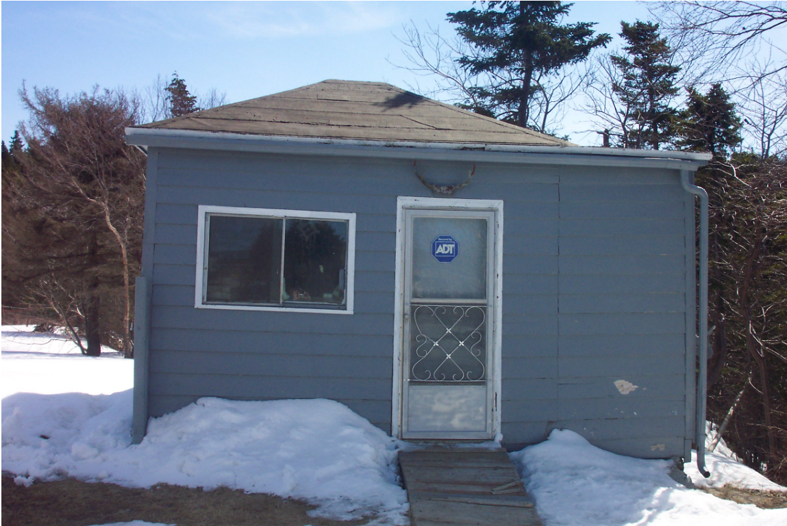
Shed at 10 Dunn's Lane, 2005.
