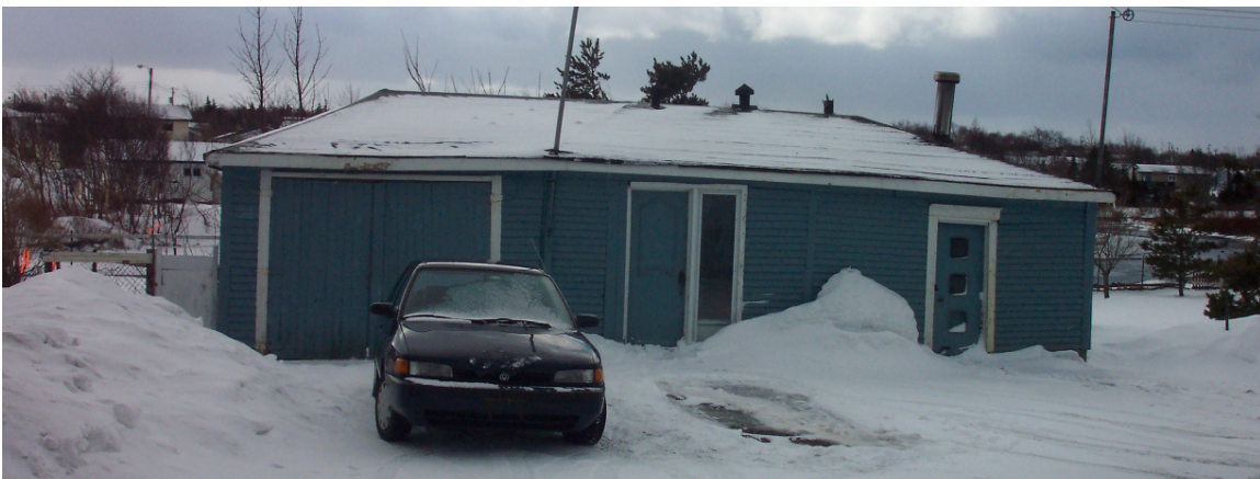
Garage/shed, 813-815 Topsail Road (February, 2005).
