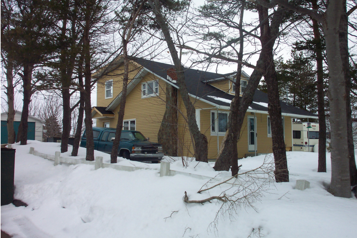
26 Park Avenue, March, 2005. Note second floor addition, new windows and vinyl siding.
