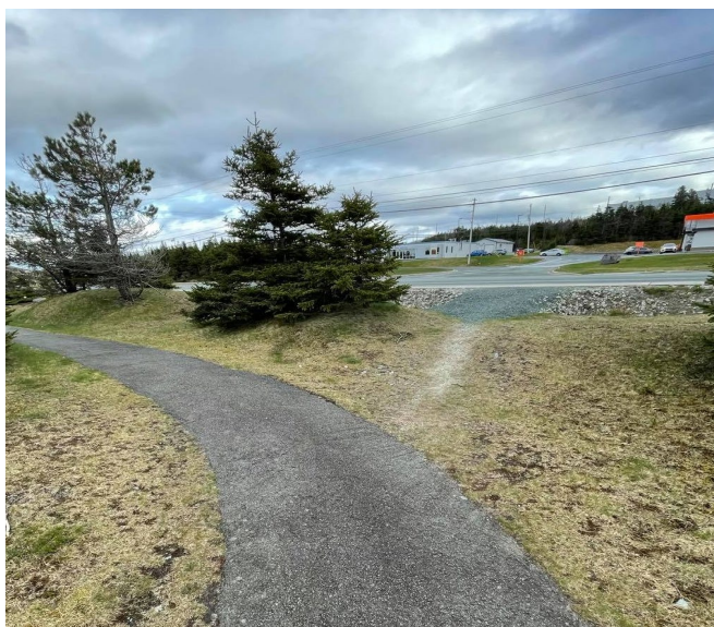
Figure 10: Asphalt trail leaving Power's Pond area near Old Placentia Road ends abruptly with no accessible route off trail
