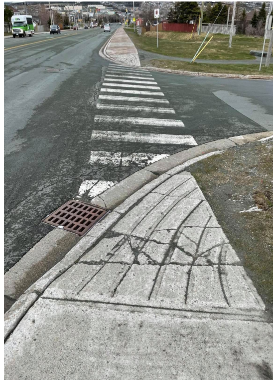
Figure 12: Sidewalks and roads along Old Placentia Road and Ruth Avenue have many cracks and bumps. Requires Tactile Attention Indicator (TAI)
