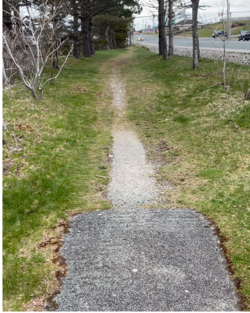
Figure 11: Asphalt trail leaving Power's Pond area near Old Placentia Road ends abruptly with no accessible route off trail
