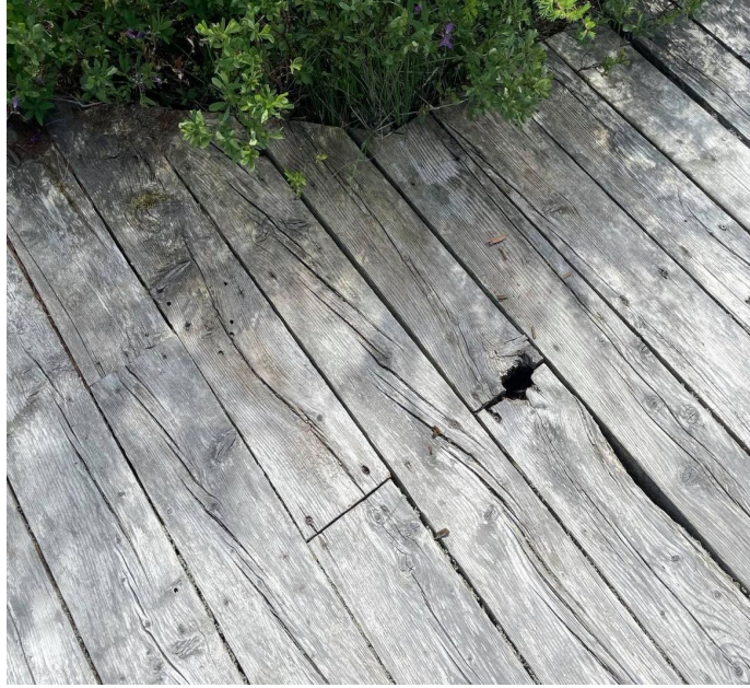
Figure 3: Broken and loose boards on boardwalk
